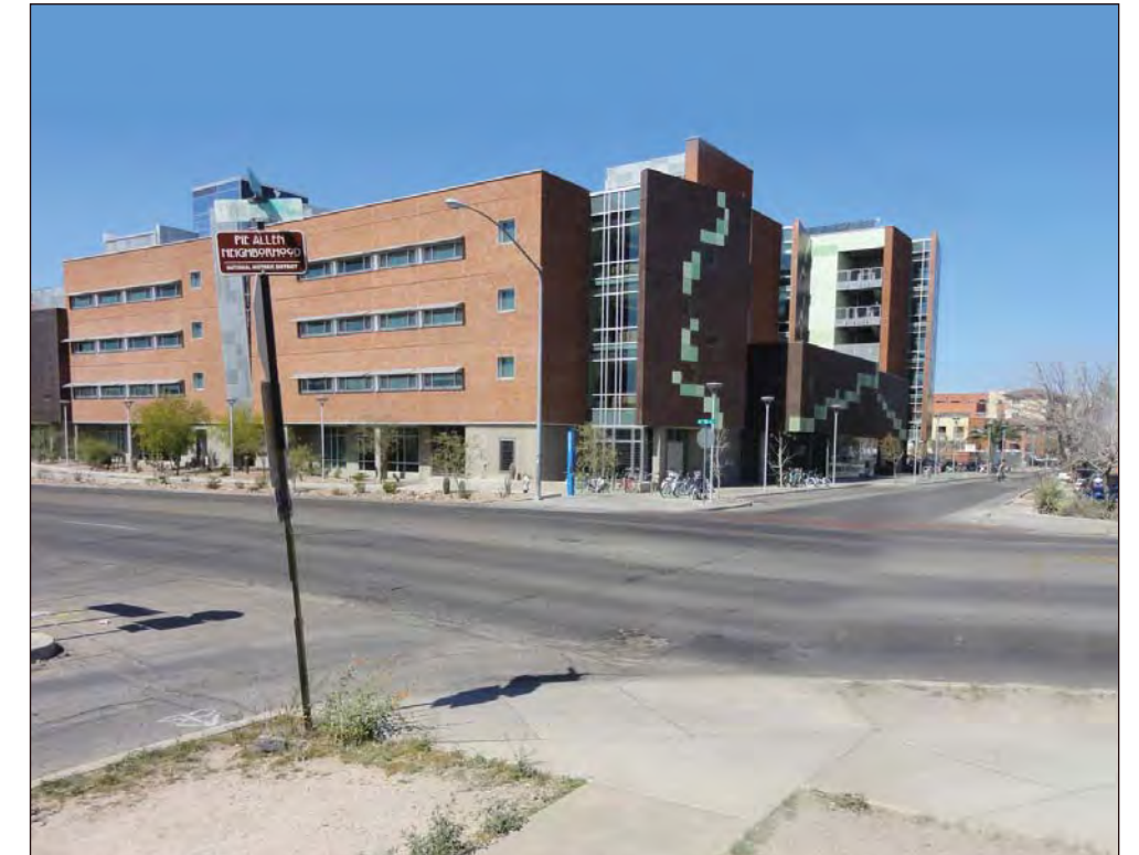
6th Street at Tyndall Avenue: Before
