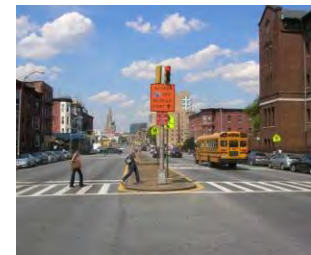
Median Refuge Island
